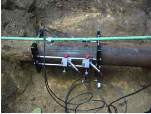
C-RL transducers installed on a 6 in (150 mm) cast iron pipe
