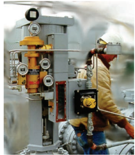
Figure 8 – Becker HPP-3 Positioner with LPDA Actuator
